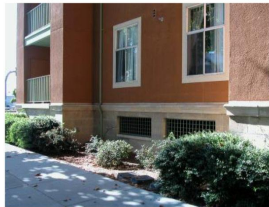
Examples of appropriately designed facades on ground level and partially underground parking levels. The parking levels have facades that are compatible with the rest of the structure and window openings with decorative metal grates to screen views into the structure: allowed
