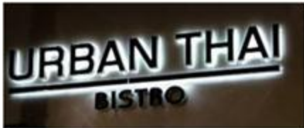
F2 Back-lighting of cut-out letters and symbols that are mounted to the wall: allowed
