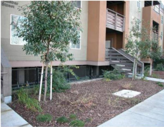
Example of inappropriately designed facade on a partially underground parking level. The building appears to “float” over the exposed parking level: prohibited
