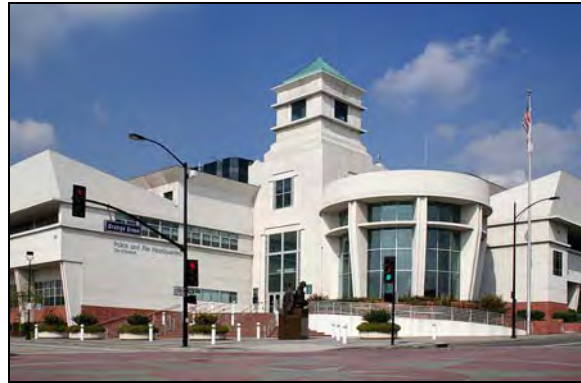
The headquarters building for both the Burbank Police and Fire Departments is located at the intersection of North Third Street and Orange Grove Avenue.
